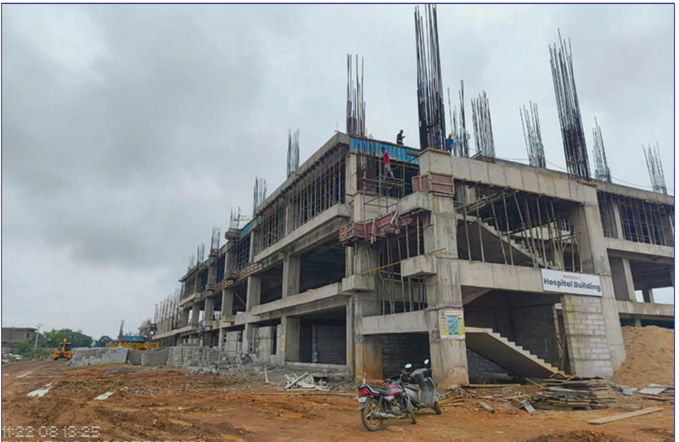
Medical College and Hospital Building, Gondia(Page 82)
