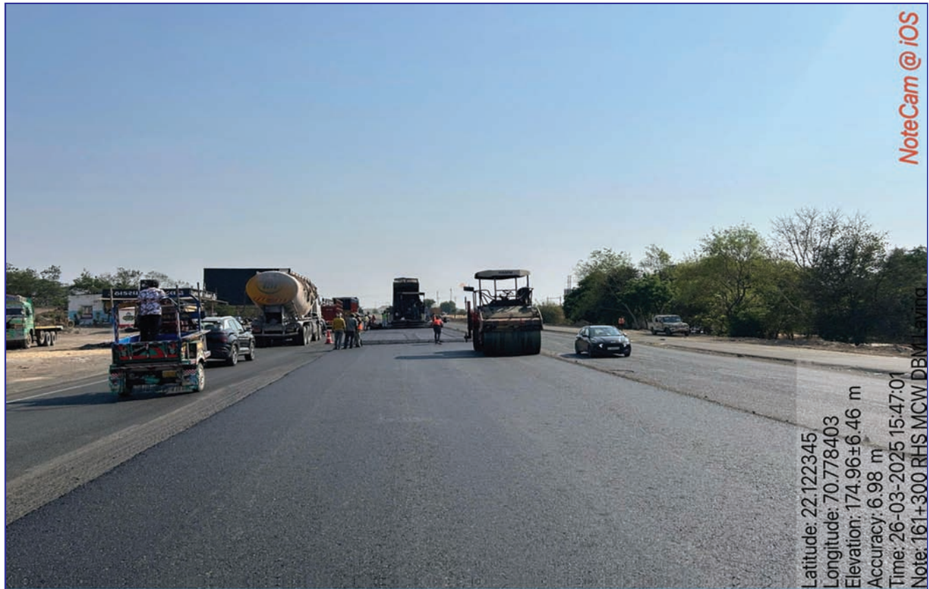
NHAI, Rajkot Widening of Four Lane to Six Lane work in progress
