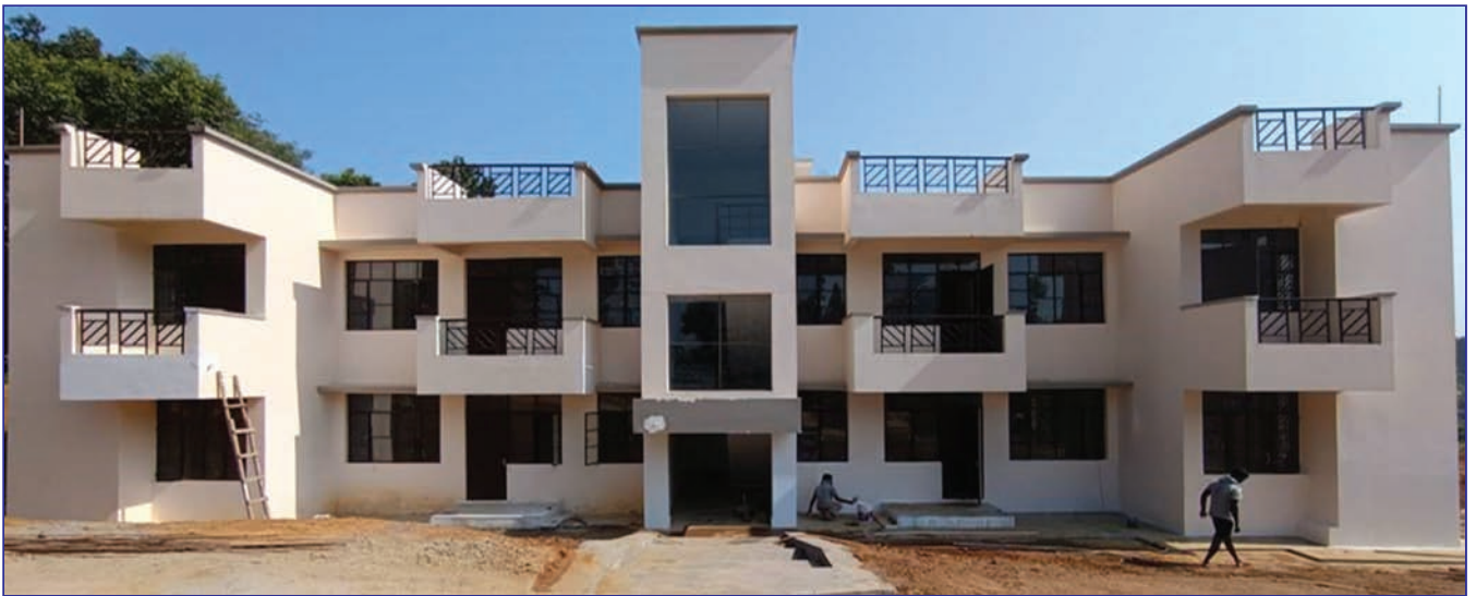
Sabroom Township Power Grid Project, Tripura
