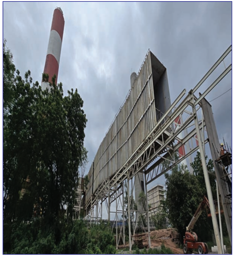
Chimney - FGD, Ramaundam
