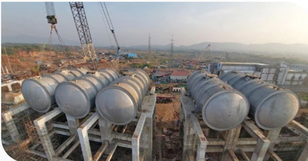
Catofin Reactors at GAIL USAR PDH-PP.
