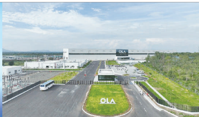
Giga factory of Ola Cell Technology Pvt. Ltd. at Krishnagiri Tamil Nadu established under PLI ACC scheme
