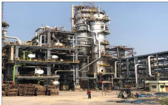
Composite Works at Ramagundam Fertilizer Complex, Telangana for RFCL
