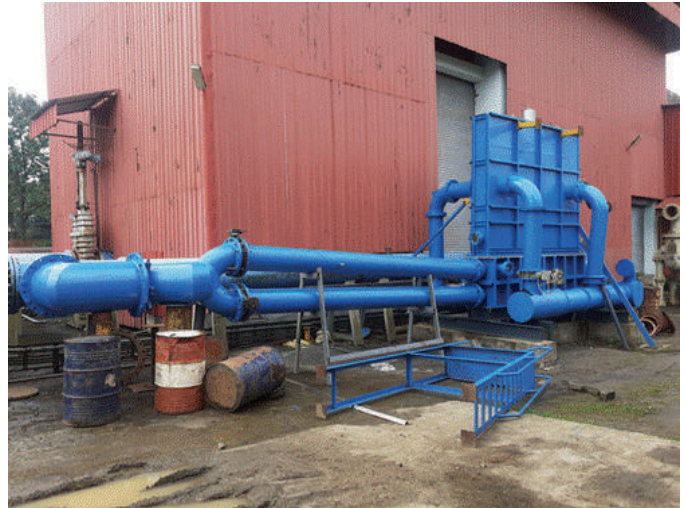
Test setup for evaluation of Hydraulic performance of slab model of purger sub assembly
