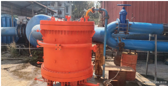
Test setup for leak rate testing
