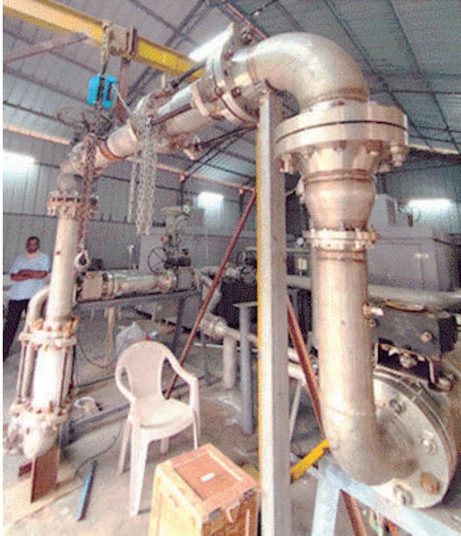
Test setup for evaluation of valve hydraulic resistance and flow Induced Vibration
