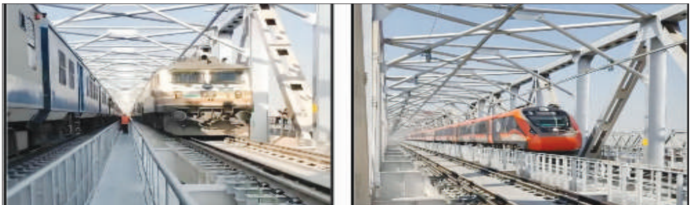
Bridge No. 1111, Ganga Bridge, Prayagraj, UP
