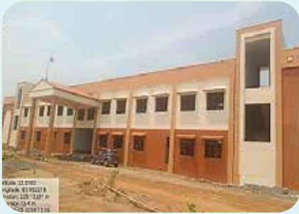
Tangarpalli (Odisha) School Building
