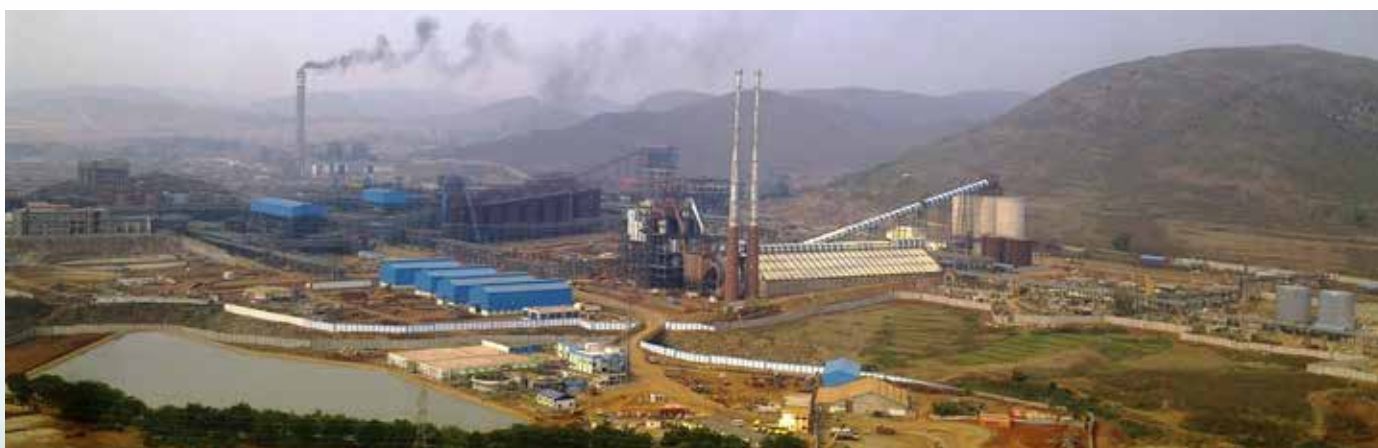
Utkal Alumina Refinery at Rayagada, Odisha
