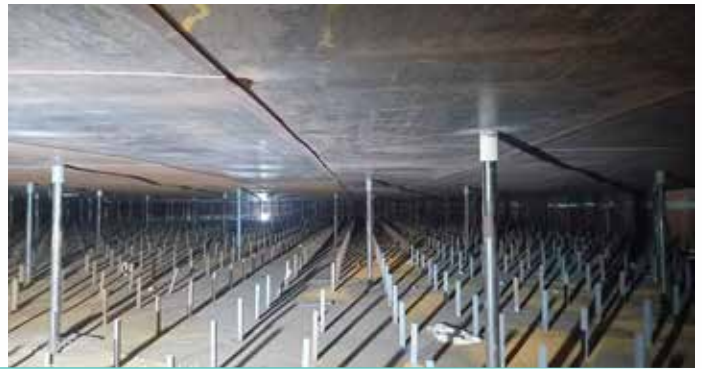
Lifting of Double Deck Roof of Floating Roof Tank by Jacking method in place of using water during construction.
