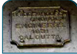
1931 Railway Bridge at Vizag
