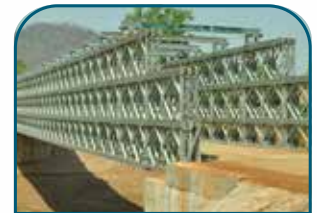
2014 Bailey Type Unit Bridges at Rayagada, Odisha
