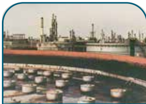
1979 Buoy Floating Roof Crude Oil Tank for Madras Refineries Ltd
