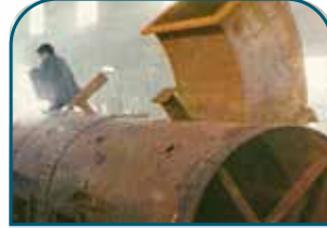
1956 Gas collecting main for Coke Oven Battery, Durgapur Steel Plant
