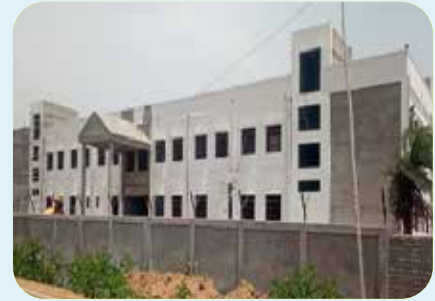
Masalia (Jharkhand) School Building
