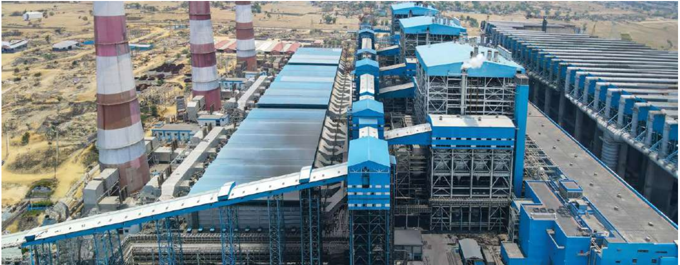
BHEL has commissioned the nation's first utility-scale thermal power plant equipped with Air Cooled Condenser (ACC) at NTPC North Karanpura Super Thermal Power Project Unit-2 (3x660 MW)
