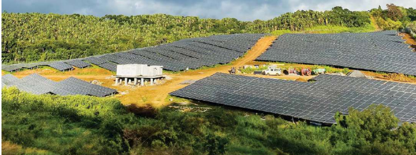
8 MW ac Tamarind Fall Solar PV Project in Henrietta, Mauritius commissioned by BHEL
