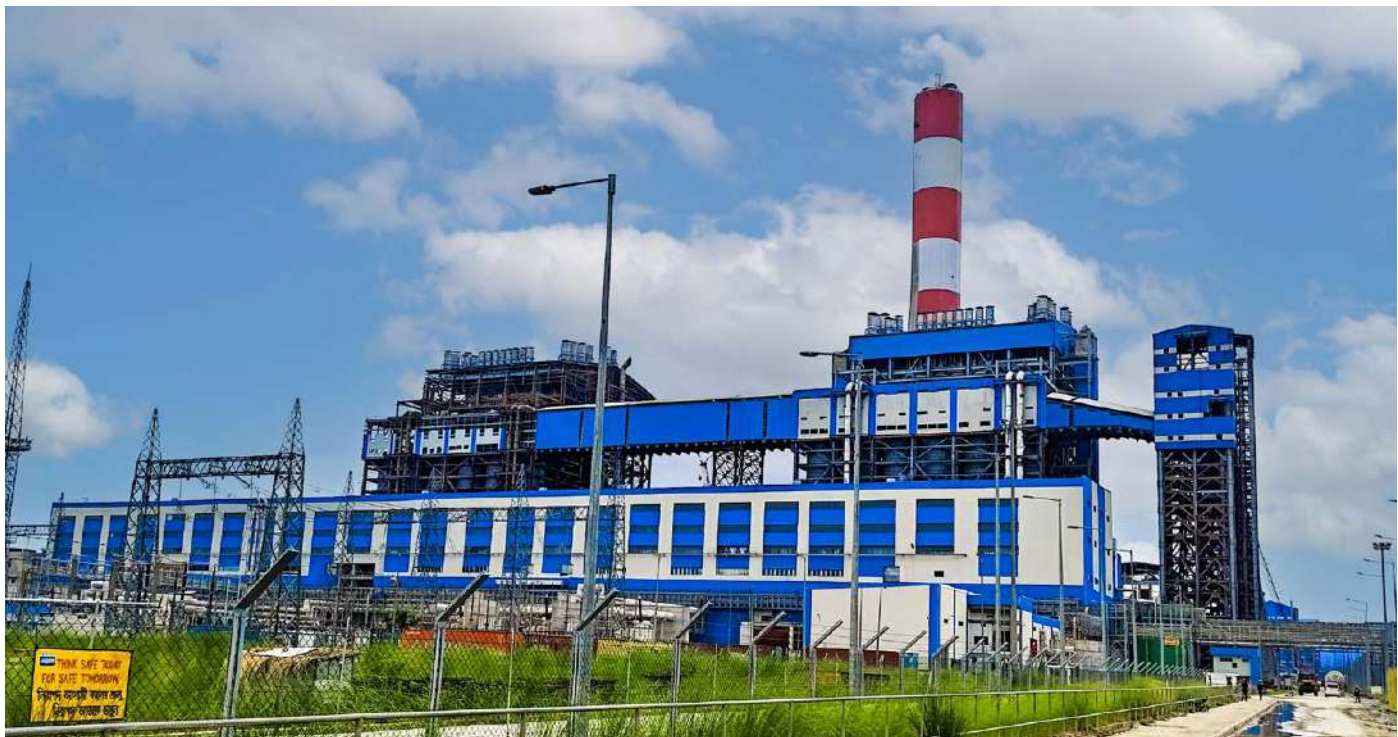
Unit 2 of 2 x 660 MW Maitree STPP, Bangladesh commissioned by BHEL
