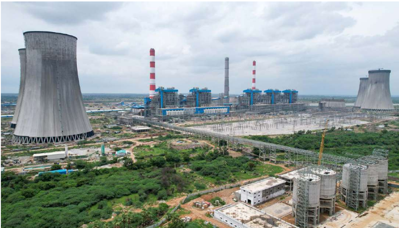
BHEL has manufactured India's first set of catalysts for Selective Catalytic Reduction for limiting NOx emissions for the 5x800 MW Yadadri Thermal Power Station in Telangana
