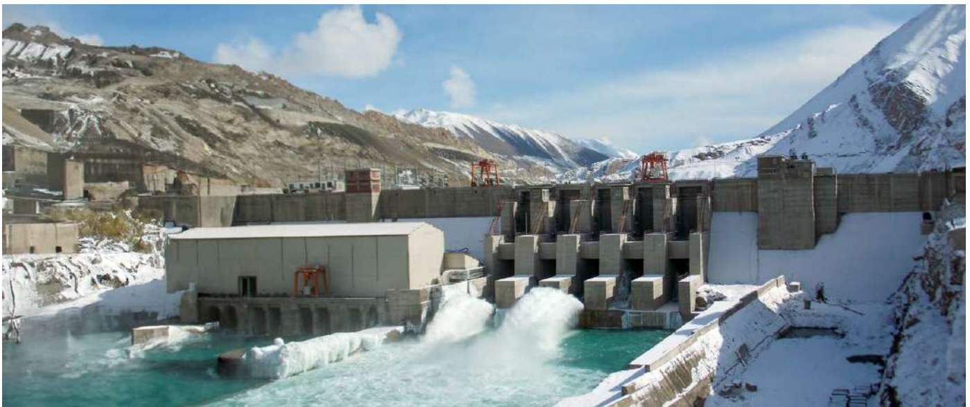
NHPC's 45 MW Nimoo Bazgo Power Station (UT of Ladakh), commissioned by BHEL (electro-mechanical works)
