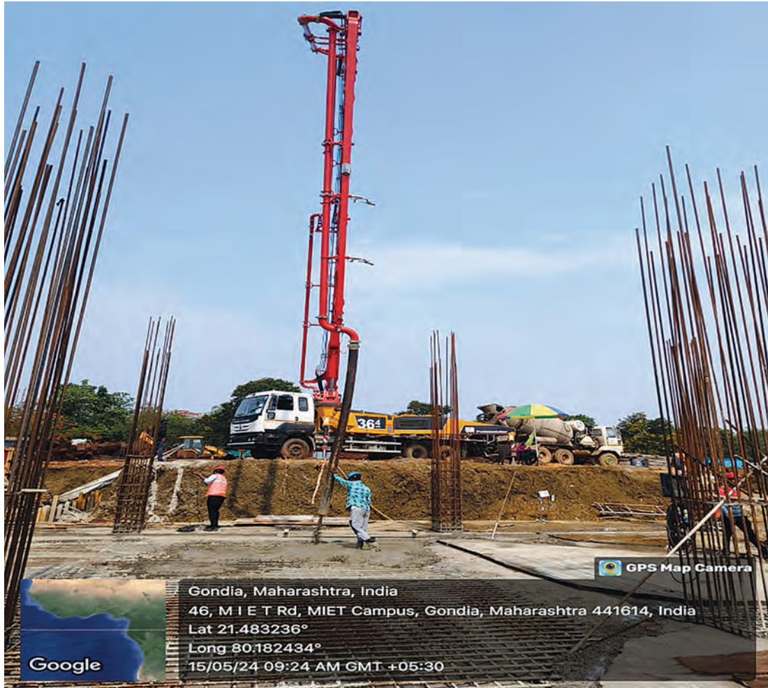
RAFT CASTING- GONDIA MEDICAL COLLEGE PROJECT
