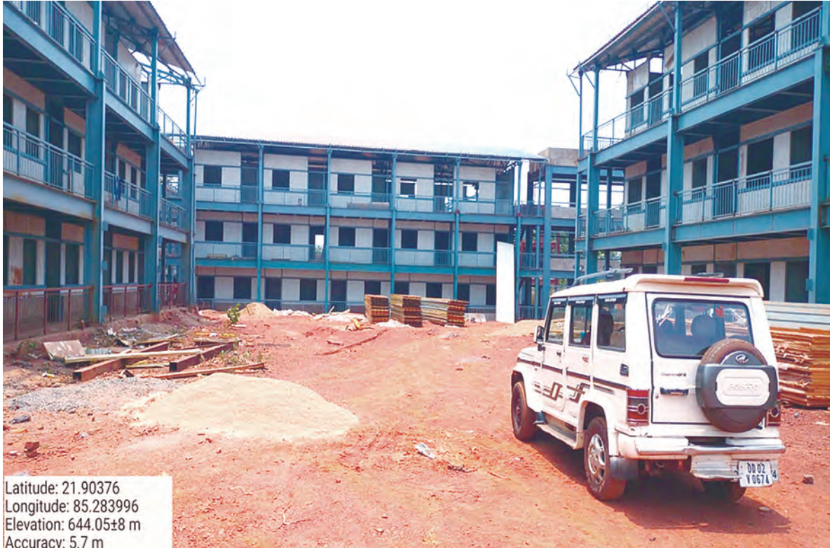
DMF 1000 LAB ACCOM & 2 Nos CREMATORIUM, SUNDARGARH, ODISHA
