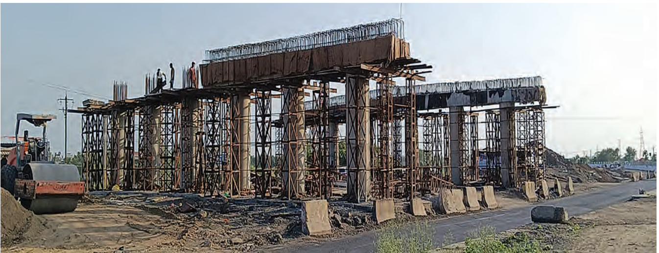
NHAI Rajkot- VUP Pier Cap work under progress
