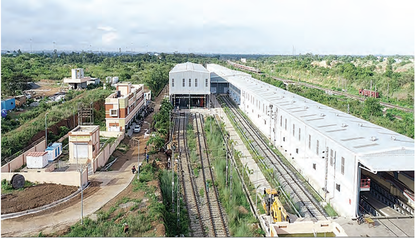
RVNL EMU CAR SHED PROJECT, KHURDA ROAD, BHUBNESHWAR, ODISHA
