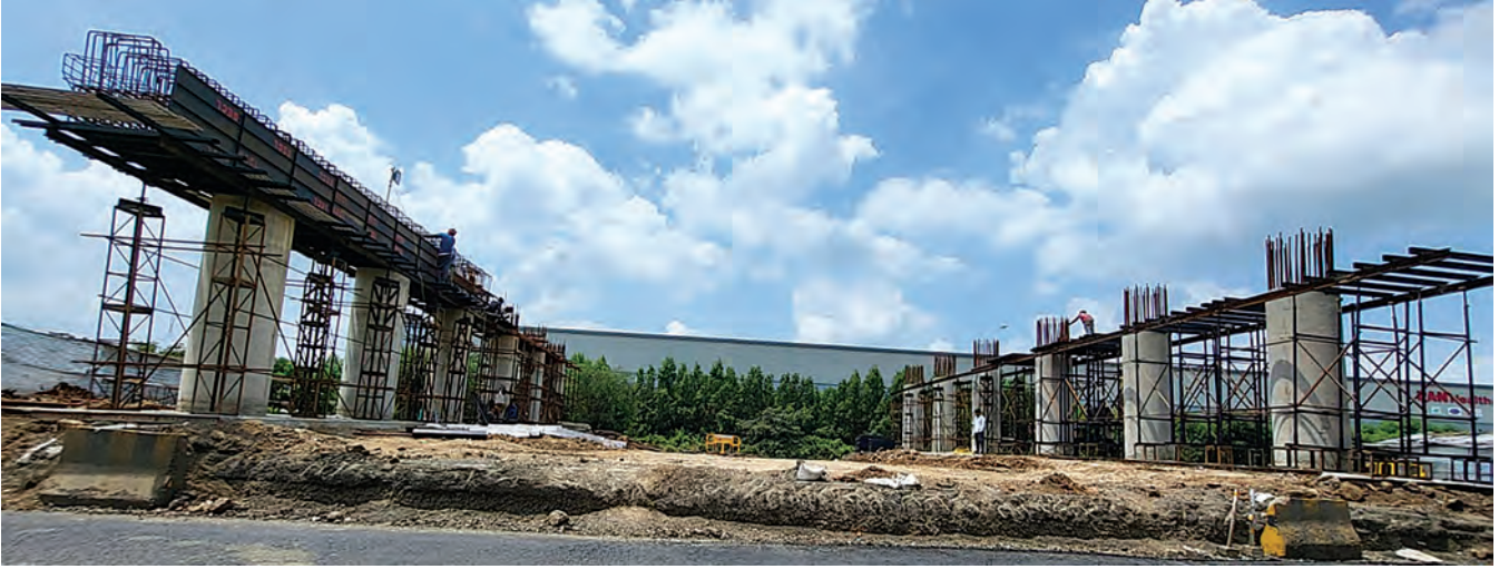
NHAI-Rajkot-Flyover work under progress
