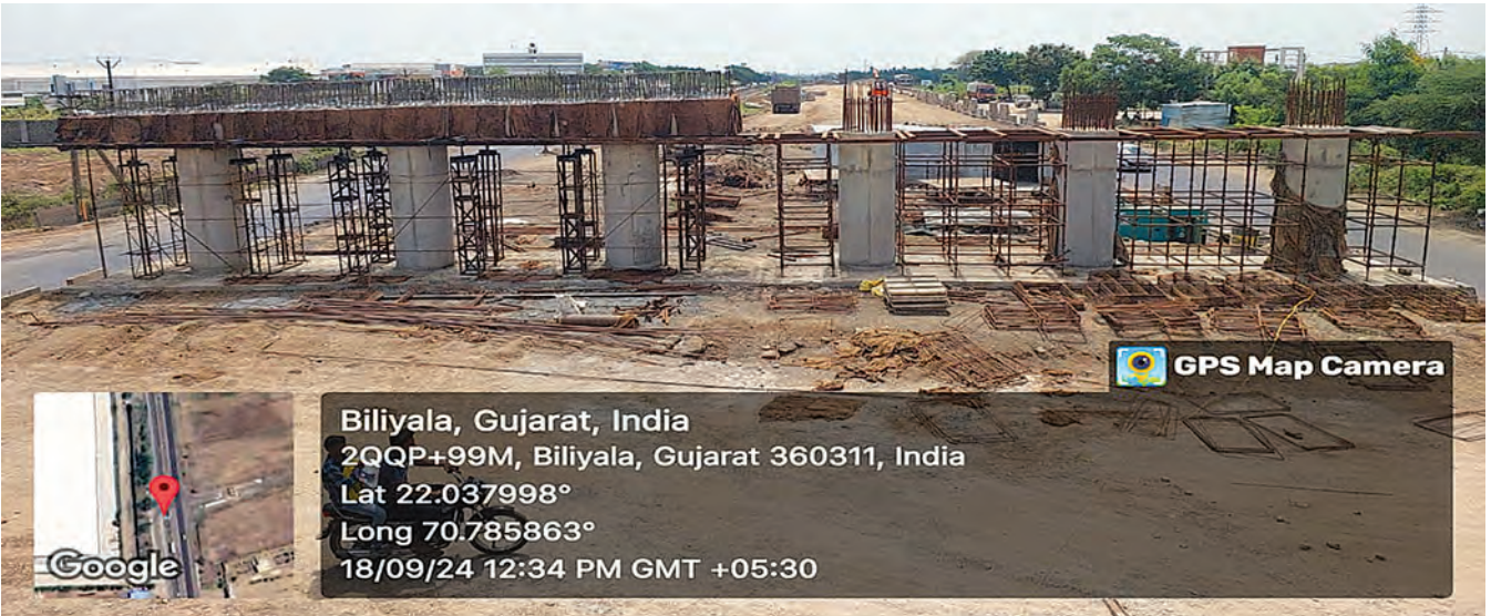
NHAI Rajkot- Flyover work under progress
