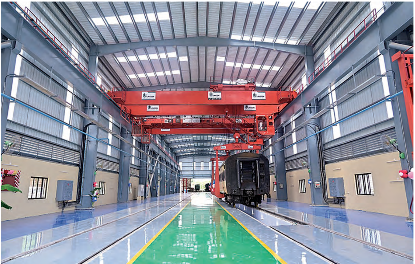
RVNL EMU CAR SHED PROJECT, KHURDA ROAD – HR BAY
