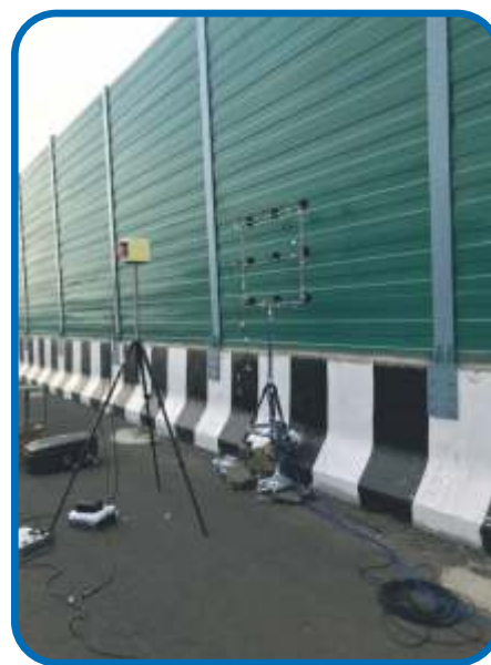
Typical Set up for in-situ Evaluation of Noise Barrier
