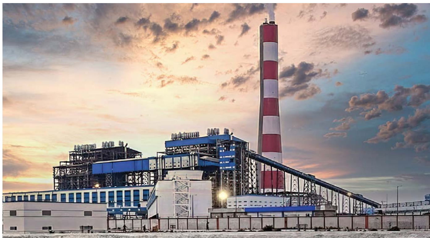
Unit 1 of 2x660 MW Maitree STPP, Bangladesh—one of the largest coal-fired power plants in Bangladesh, which commenced commercial operation, was inaugurated by Hon'ble Prime Minister of India
