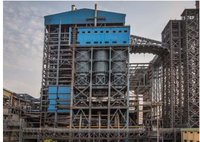
700 MW STPP executed by BHEL at Bellary, Karnataka for KPCL
