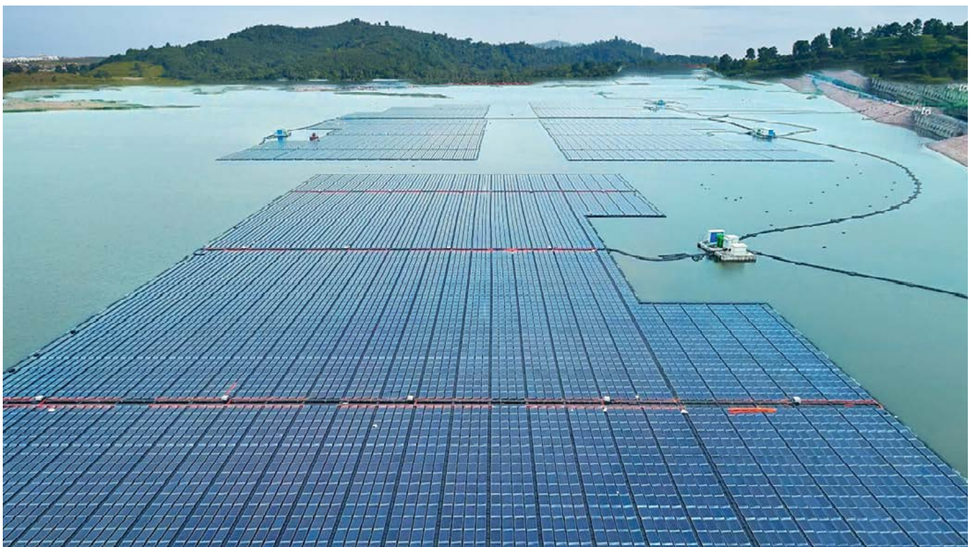
100 MW Solar PV Plant at NTPC, Ramagundam, Telangana, the largest floating solar power plant in the country, commissioned by BHEL
