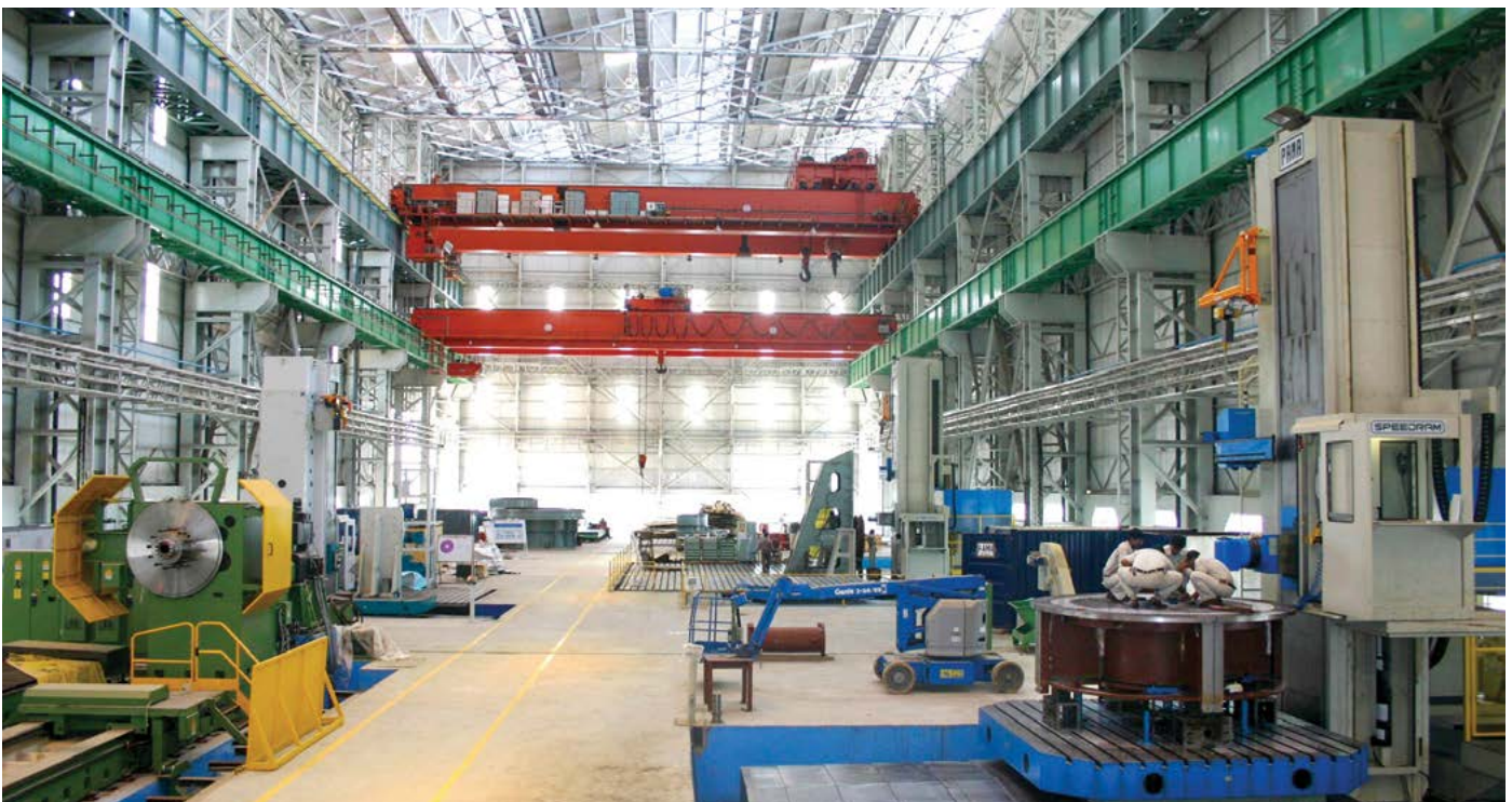
New CNC Hydro Block set-up in Bhopal plant, for augmenting hydro manufacturing capacities
