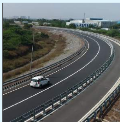
HIGH SPEED TRACK AT GARC
