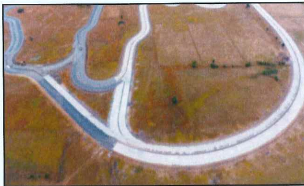
Gravel and Off road Track
