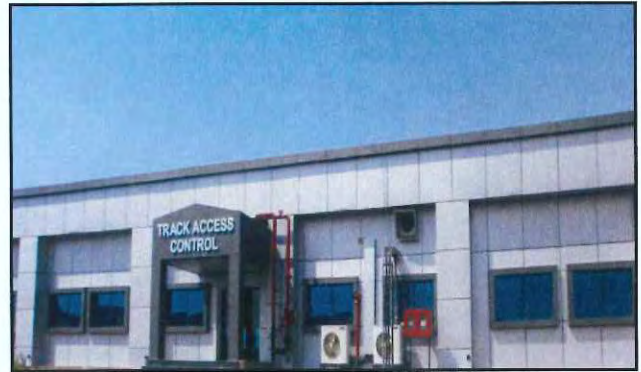
Track Access control
