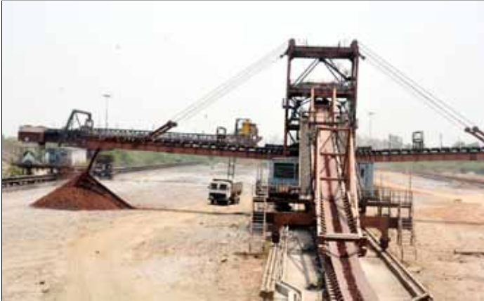
Commissioning of Wagon Tippler Route at Bhilai Steel Plant
