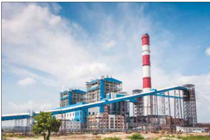
BHEL forayed into power generation with its JV project, 2x800 MW Yeramarus TPS
