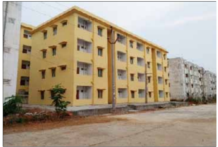
Flats constructed by BHEL at Vizag for Hud-Hud affected people.
