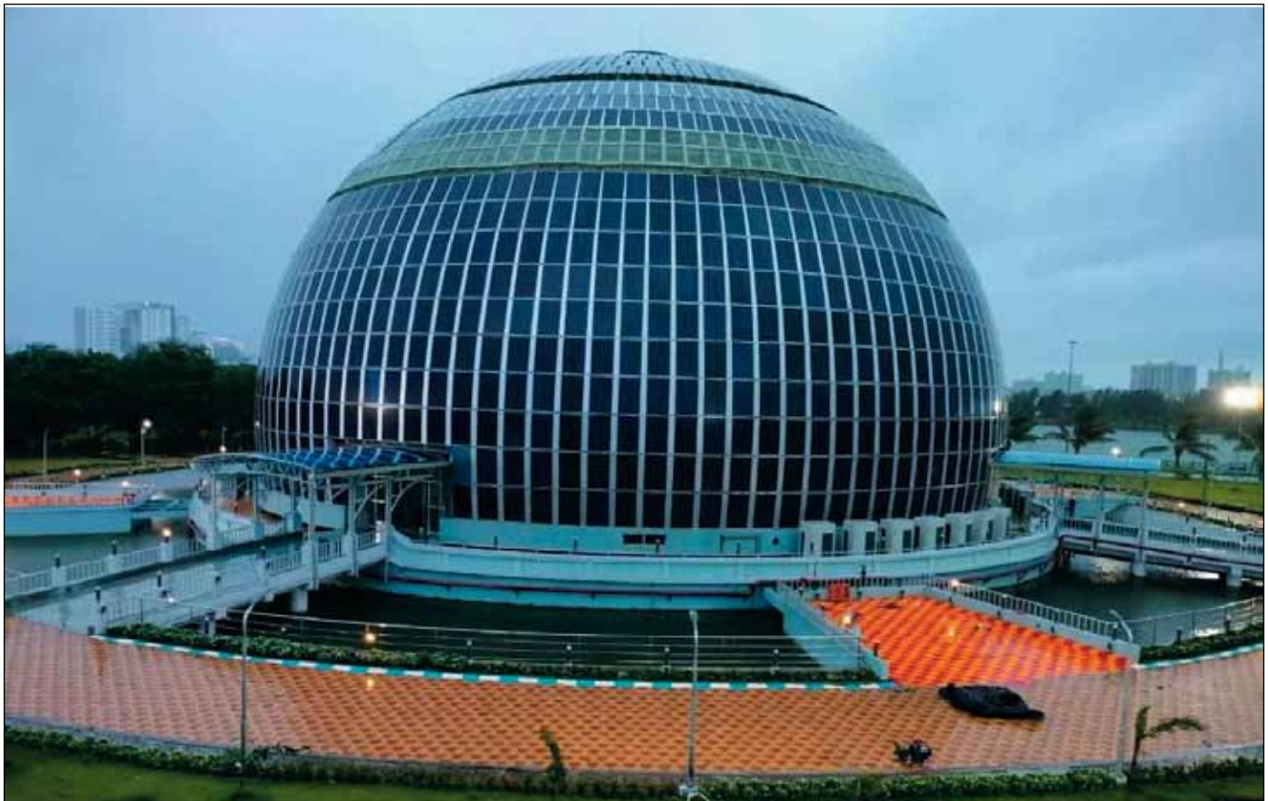
Construction of Solar Dome at Eco-Park, Kolkata for West Bengal State Electricity Distribution Co. Ltd., Govt. of West Bengal
