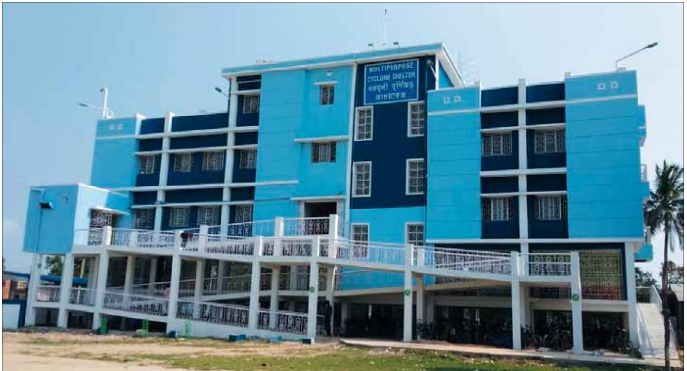
Construction of 98 Nos. Multipurpose Cyclone Shelters under National Cyclone Risk Mitigation Project for Department of Disaster Management, Govt. of West Bengal
