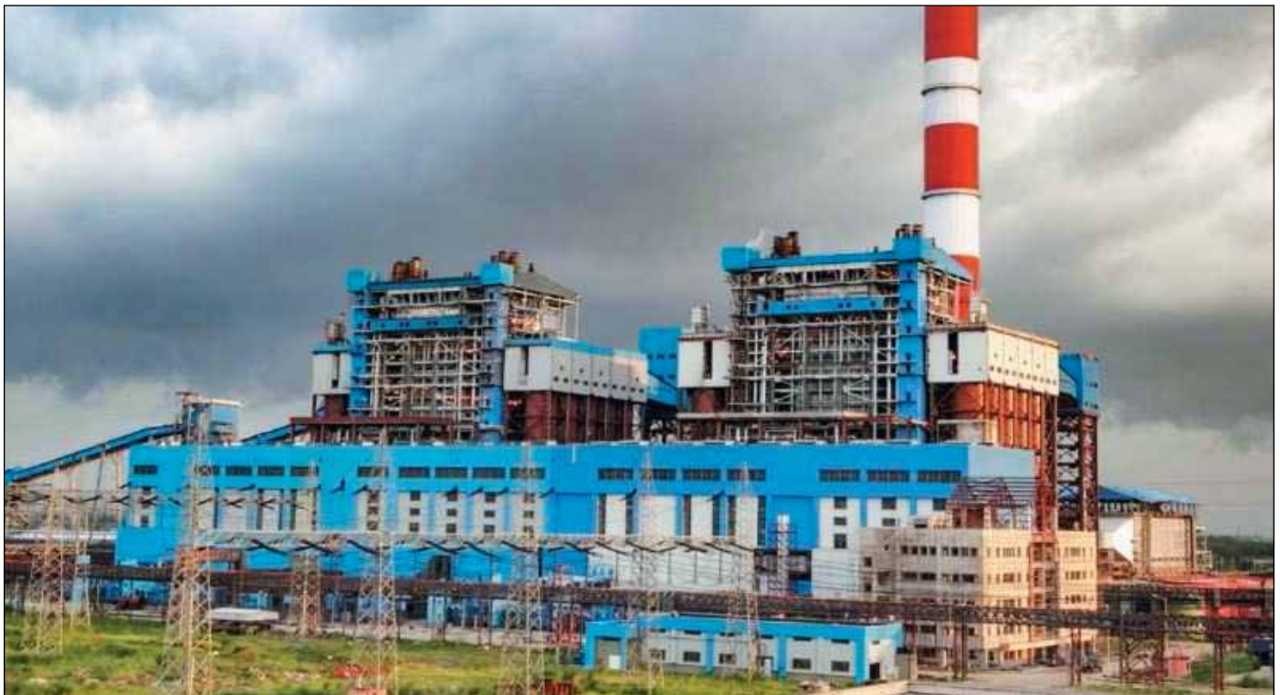
Power Block Unit for 2x500 MW Unit # 1 & 2 at Durgapur Steel Thermal Power Station of DVC at Andal, West Bengal
