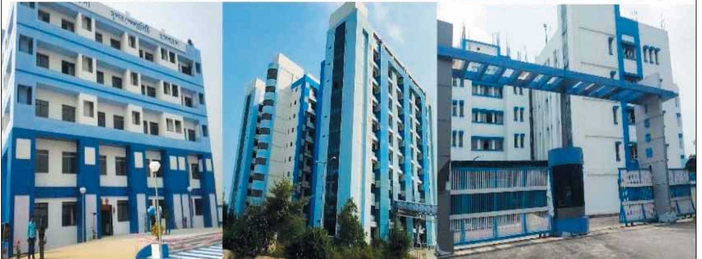
Super Speciality Hospitals for West Bengal Medical Services Corpn Ltd.at Islampur and Onda, West Bengal
