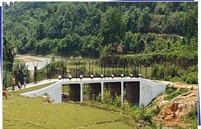
BOX CULVERT, ROAD & FENCE, TRIPURA
