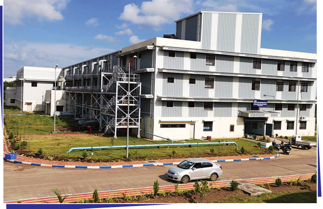
HAL NASIK PROJECT- MAA BUILDING
