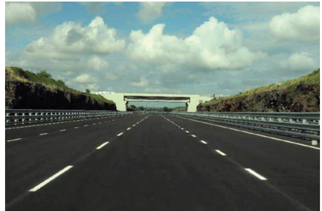
HST- Southern Straight Main Pavement
