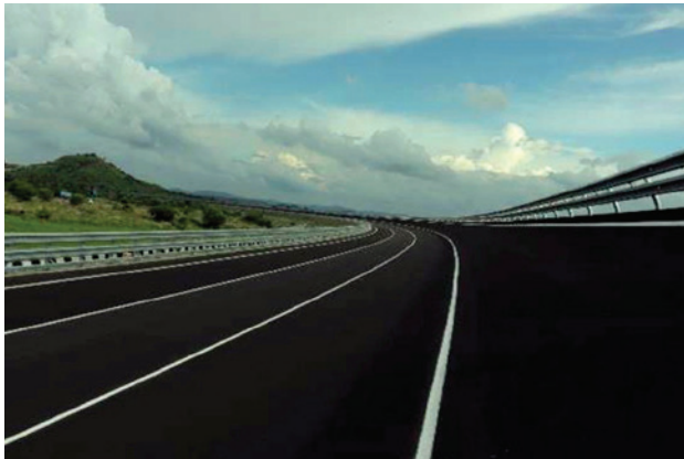
HST-Western Parabola Main Pavement
