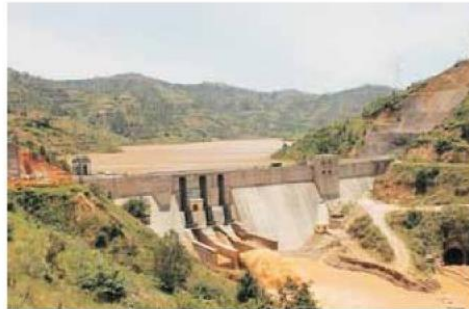
28 MW Nyaborango Hydroelectric Plant, Rwanda
