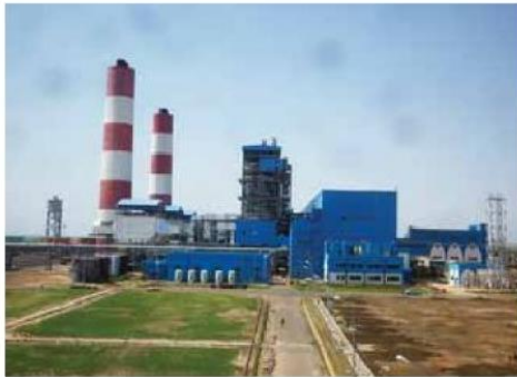
500 MW Kosti Thermal Power Station, Sudan
