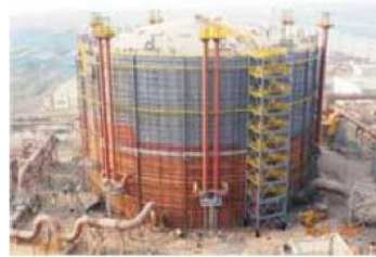
Construction of Gas Holder at IISCO, Burnpur
