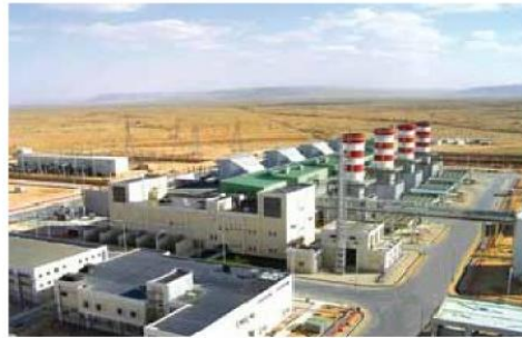
600 MW Western Mountain Gas Power Plant, Libya
