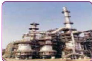
Turnkey Construction of 3 Nos. Non-IFP Heater at IOCL Panipat
