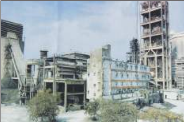
Tandur Plant (Andhra Pradesh), CCI
