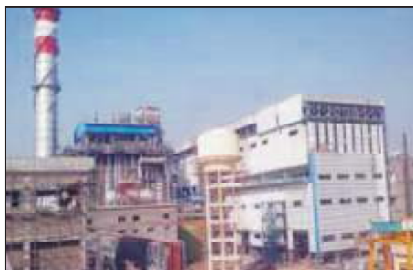
351 MW CCPP commissioned by BHEL for GSEGL, Hazira
