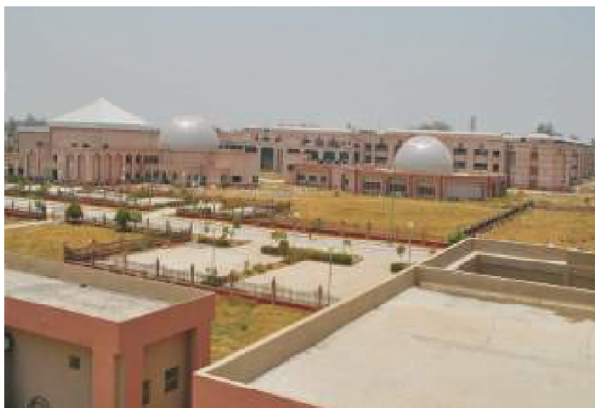
CDRI Campus, Lucknow- Constructed by EPI
