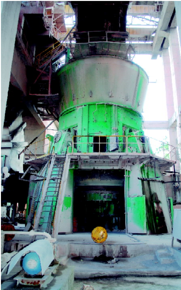
Upgradation work at Tandur Unit
