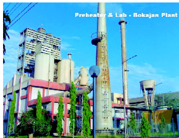
View of Bokajan Plant
