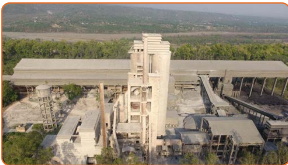
Rajban Unit Situated in Sirmaur District, State- Himachal Pradesh
