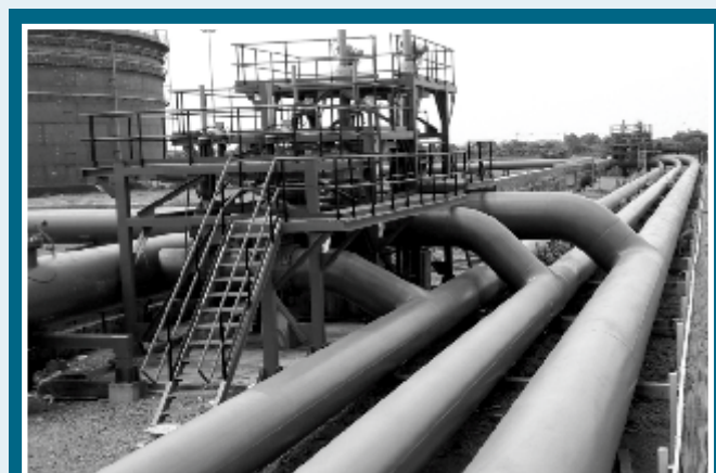
Mechanical Work at BORL Bina Terminal
