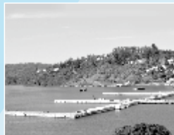
Piling & Marine Work
