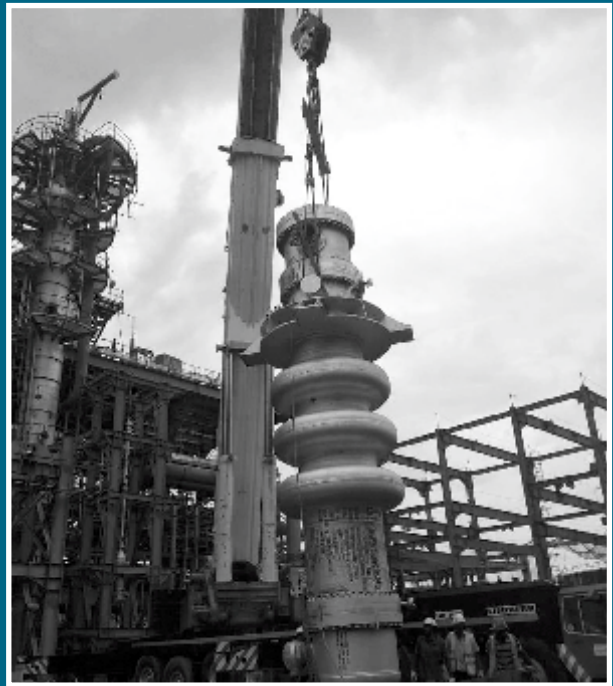
Equipment erection at FCC - DGS unit at CPCL Chennai
