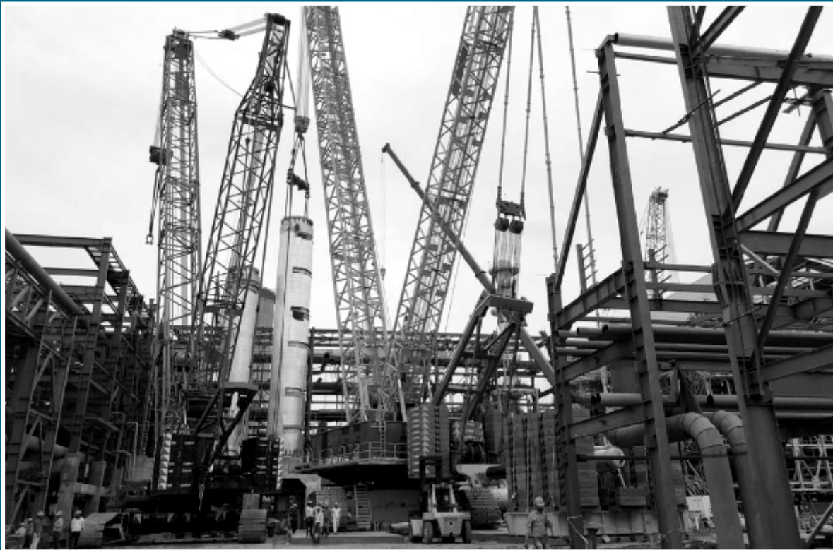
Ammonia Converter-1 Wt 700 MT being erected at RFCL Ramagundam
