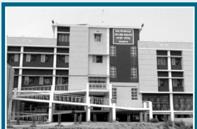
Construction on Multipurpose Cyclone Shelter under NCRMP-II at various coastal areas of West Bengal
