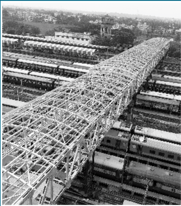
162m long Foot Over Bridge at Santragachi Station for South Eastern Railway
