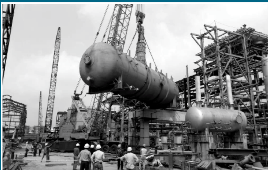
103T Vessel erection being carried out in ARU-SWS at IOCL, Haldia
