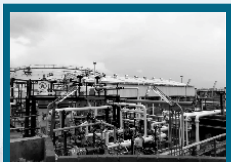
Composite Works for Mumbai Aviation Fuel Farm Facility
