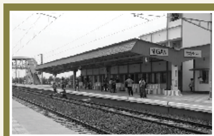
Platforms, Linking of Track, Points & Crossings and other Ancillary Works from Balgona to Katwa in West Bengal for Eastern Railway
