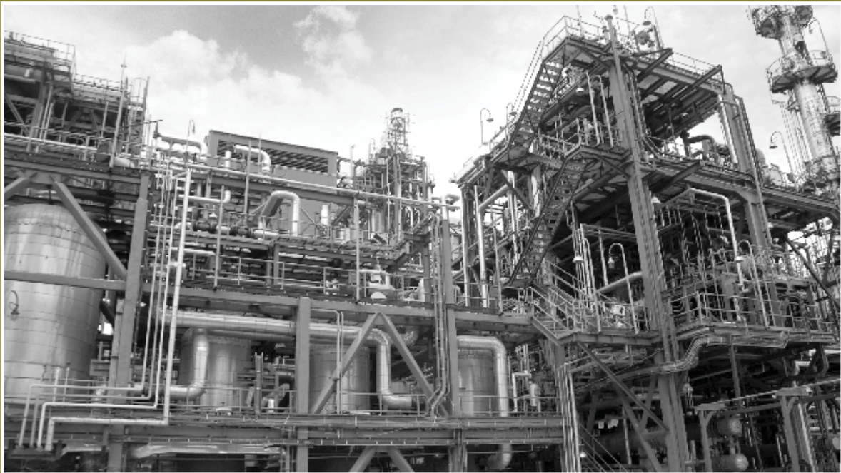
Integrated Refinery Expansion Project (IREP) for BPCL at Kochi
