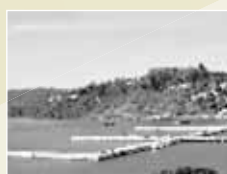
Piling & Marine Work
