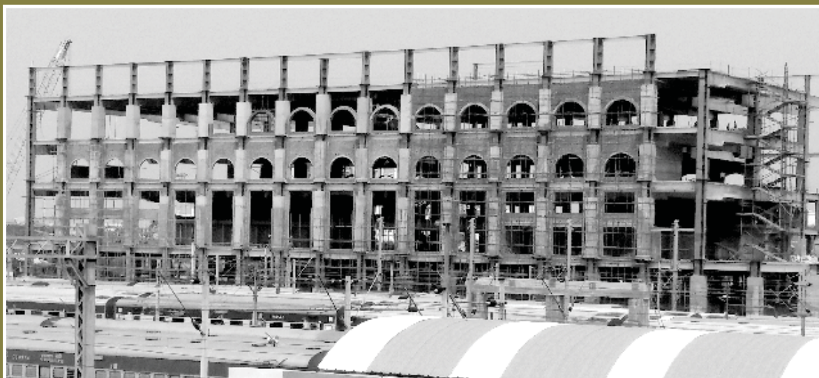
Station Development Work of Santragachi Station for South Eastern Railway
