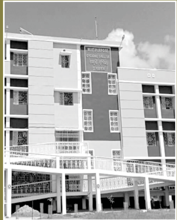
Construction of Multipurpose Cyclone Shelter, Under NCRMP - II at various coastal areas of West Bengal
