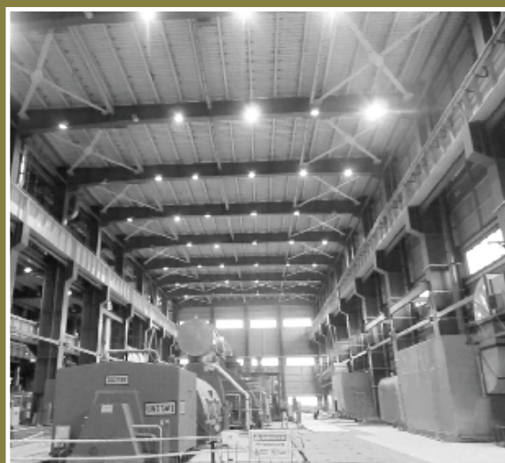
Unit-I TG Floor at NTPC Gadarwara
