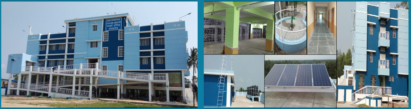
Construction of Multipurpose Cyclone Shelters (MPC) under National Cyclone Risk Mitigation Project (NCRMP-II) at Block Basanti (12 MPC), Sagar (10 MPC), Kakdwip (9 MPC), Namkhana (10 MPC), Patharpratima (12 MPC), Mathurapur-II (5 MPC) & Kultali (6 MPC) in Dist. South 24 Parganas, Block Hasnabad (3 MPC) & Minakha (4 MPC)
