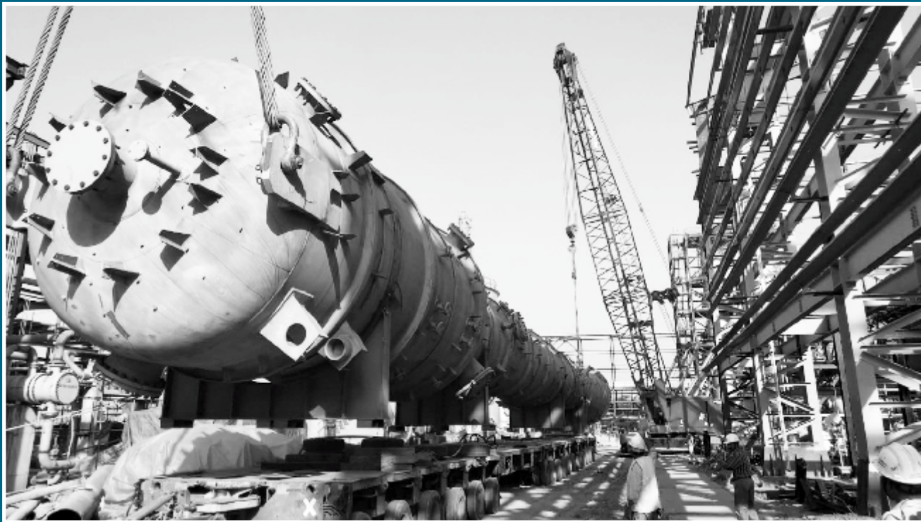
Tankage Work for Bina Despatch Terminal of Bharat Petroleum Corporation Ltd.
