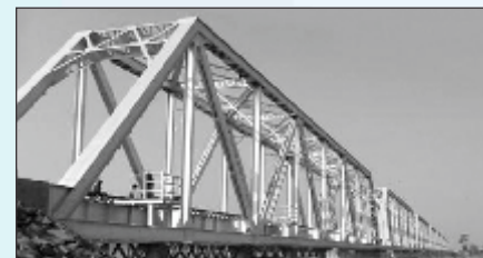
Railway Bridge Girder
