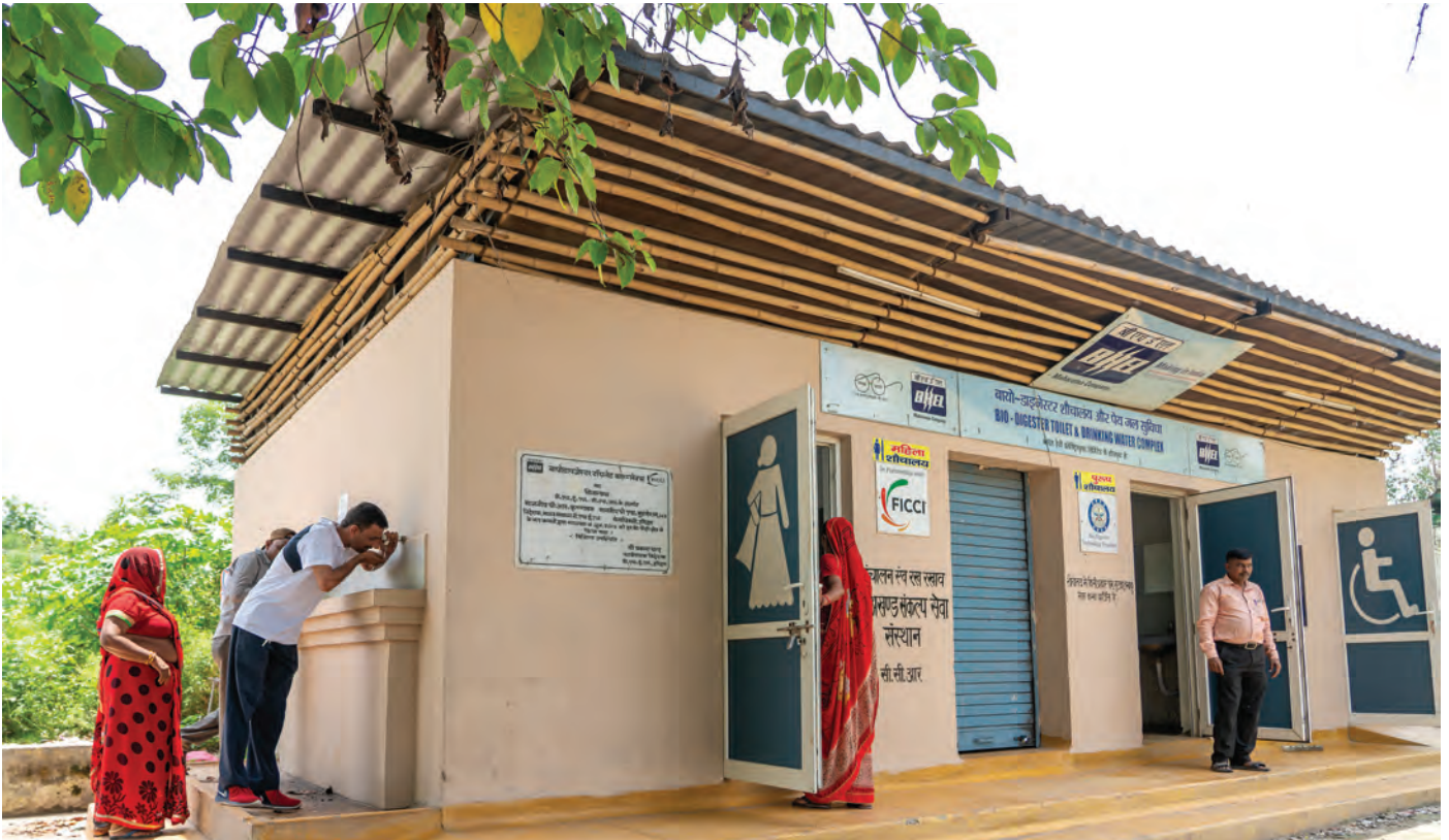
Bio-digester toilets on the banks of river Ganga near Haridwar & Rishikesh, installed by BHEL
