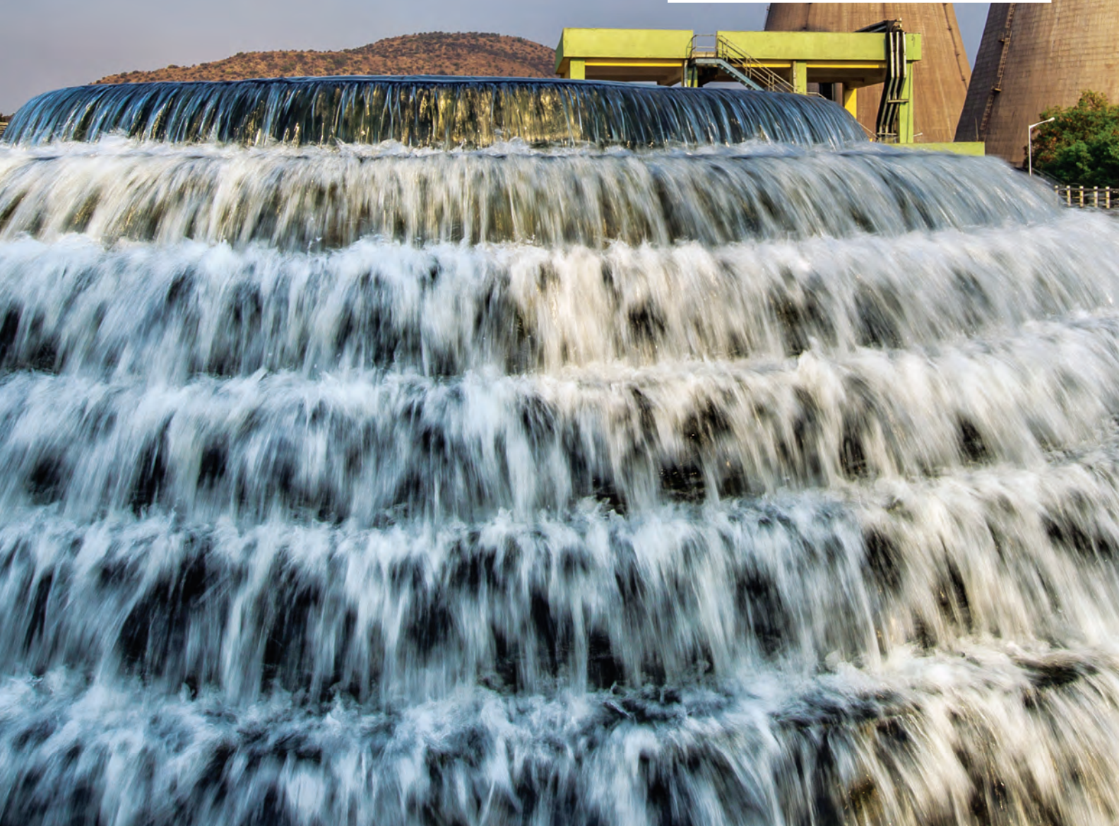
Raw Water Treatment Plant at OPaL Dahej
