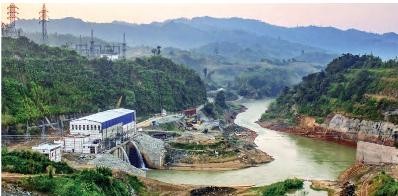
Power house of 2x30 MW Tuirial Hydro Electric Project (HEP) commissioned by BHEL in Mizoram
