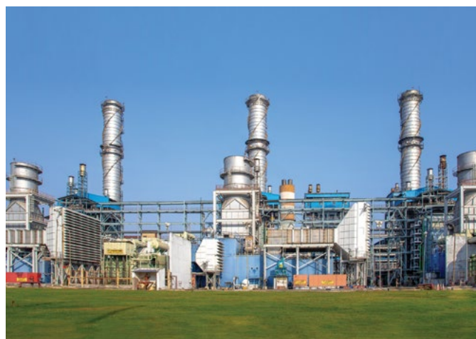
BHEL has made an entry into the downstream oil & gas process package business by securing an order for setting up 525 TPD Sulphur Recovery Unit at IOCL's Paradip Refinery in Odisha
