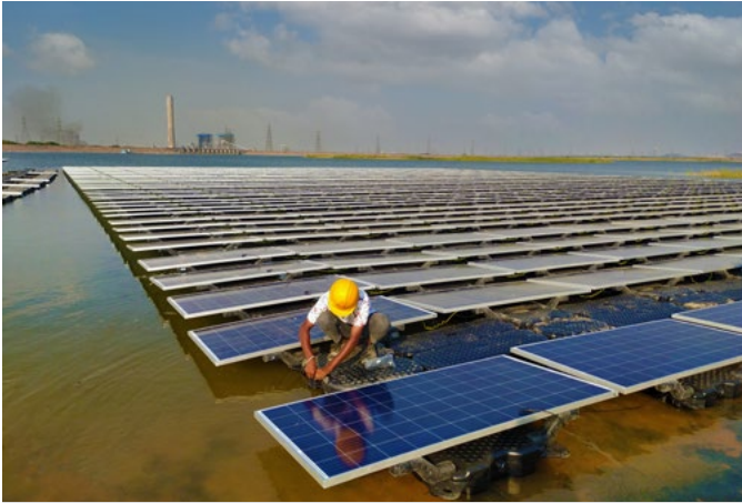
5MW AC Grid Connected Floating Solar PV project at Sagardighi Thermal Power Plant commissioned by BHEL
