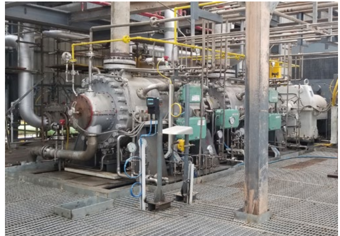
Net Gas compressor package of BPCL Kochi MS block project commissioned by BHEL
