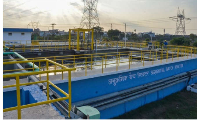
BHEL has set up a 7 MLD capacity Sewage Treatment Plant (STP) based on Sequential Batch Reactor technology, for its factory premises and suburb at Haridwar
