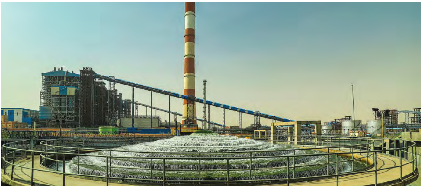
2x660 MW super critical power plant under commissioning by BHEL at Suratgarh, Rajasthan
