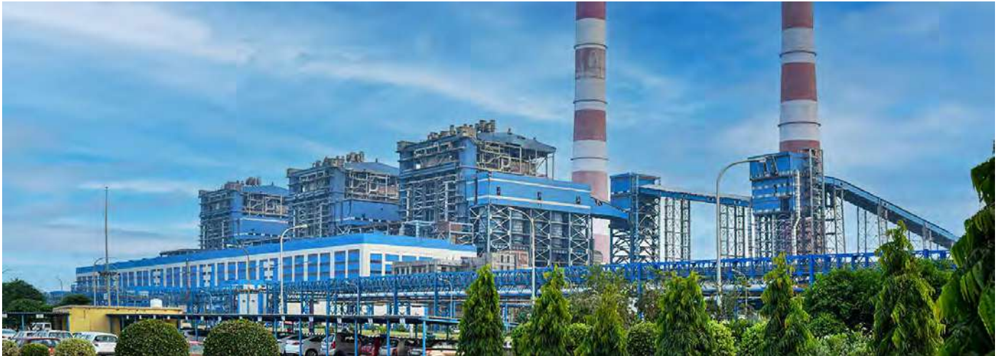
BHEL appreciated by customer (NTPC Ltd.) for best safety performance at 660 MW NPGCL Nabinagar
