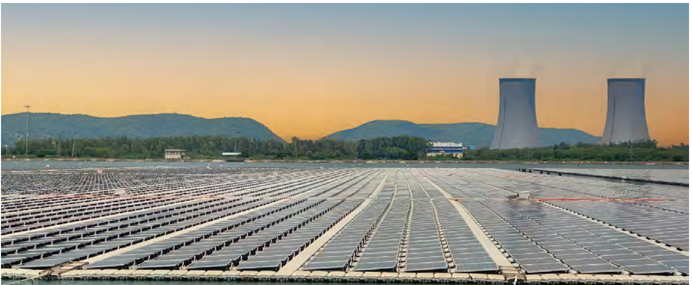
100 MW NTPC Ramagundam floating Solar PV- country's largest floating solar SPV plant, commissioned by BHEL
