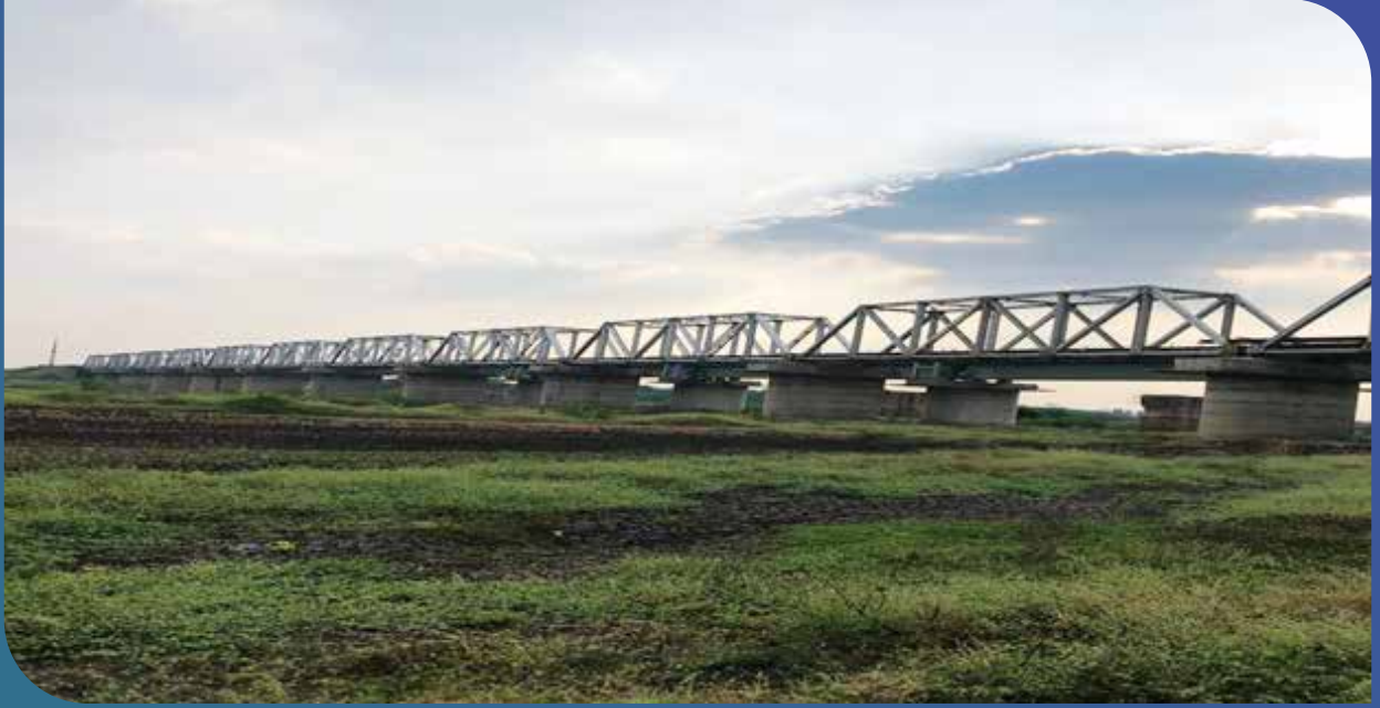
Bridge under completion at Gadag-Hotgi, Karnataka.
