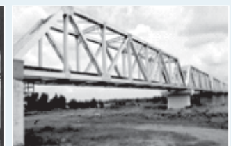
Railway Bridge Girders
