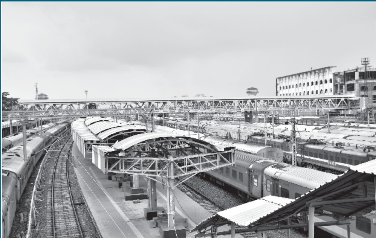
Station Development Work of Santragachi Station for South Eastern Railway
