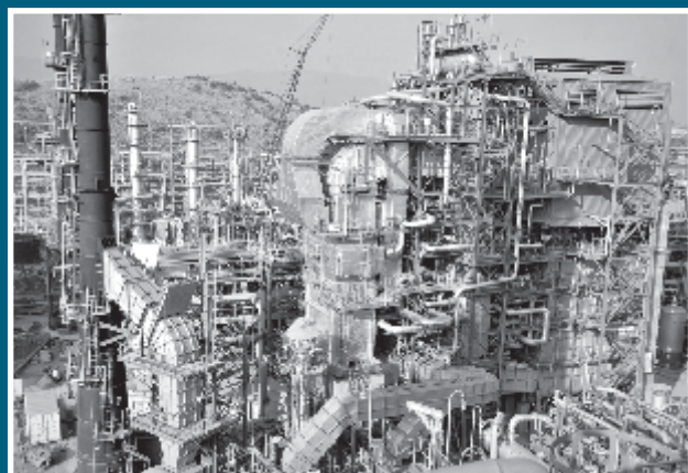
TGTU Unit at Hindustan Petroleum Corpn. Ltd. Vizag Refinery
