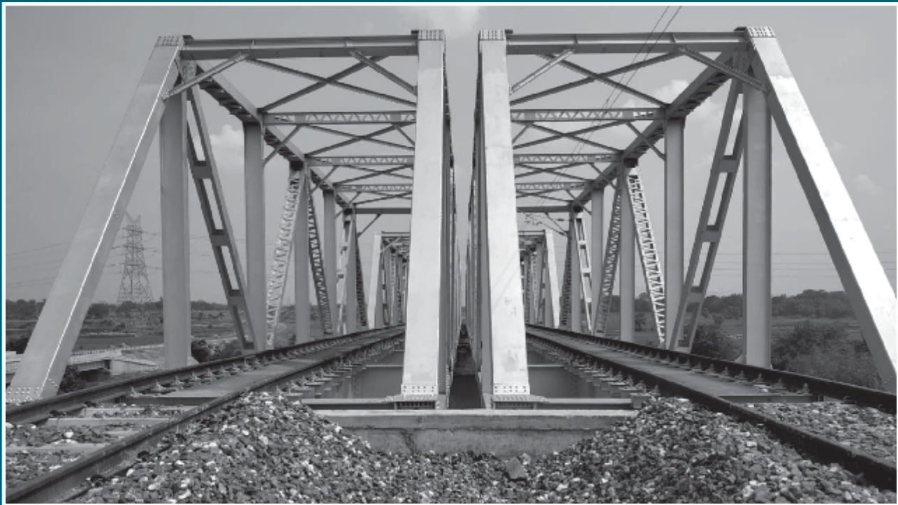
3x2, 30.5 m open web through girder rail bridge over Uthala River at railway siding project of DVC for RITES Ltd. at Raghunathpur
