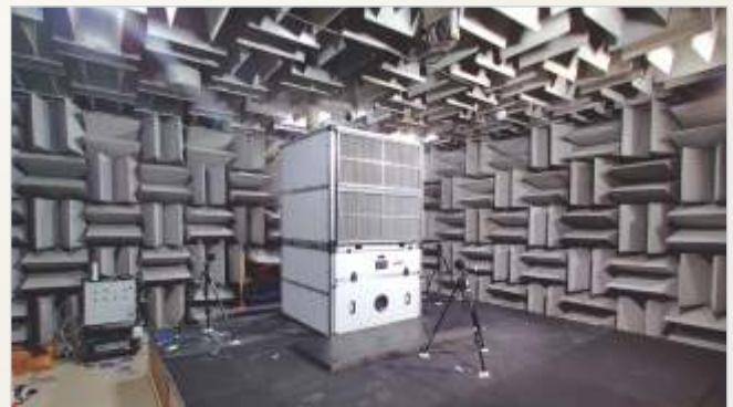
Noise Reduction of Air Handling Unit
