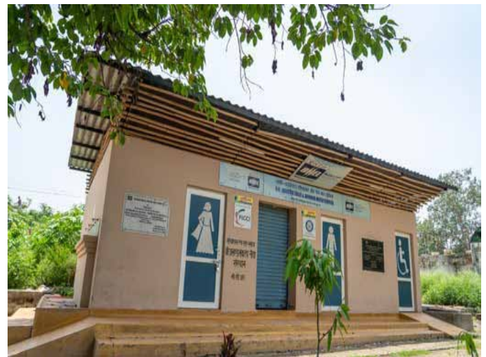
Bio-digester toilets on the banks of river Ganga near Haridwar & Rishikesh installed by BHEL
