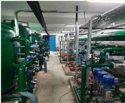
Track Irrigation system (Sump & Pump house)
