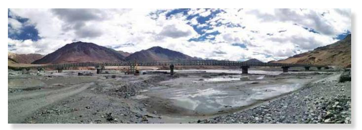
Manufacture, supply, erection and commissioning of 1400ft. (10x140') long Bailey Bridge of carriage way of 4.25m on Darbuk Shyok-Daulat Begh Oldie Road in Leh, for the Border Road Organisation
