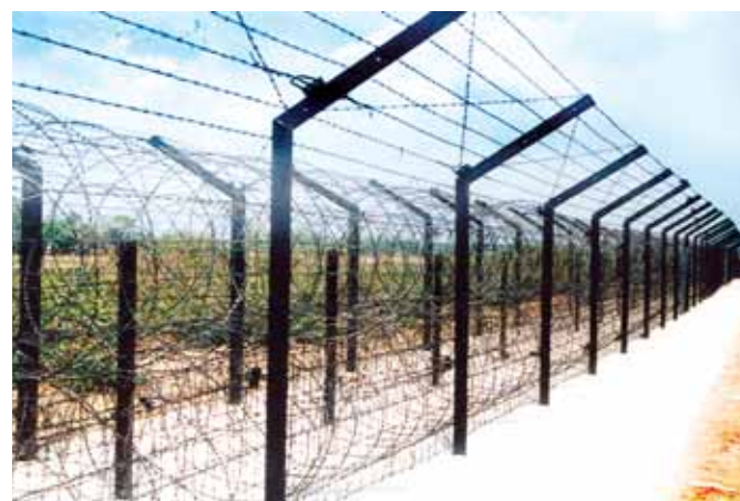
EPI executed Indo-Bangladesh Border Fencing, Tripura
