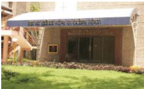
BHEL's Centre of Excellence for Intelligent Machines
