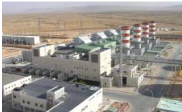
600 MW Gas turbine-based Western Mountain power project in Libya, set up by BHEL on turnkey basis
