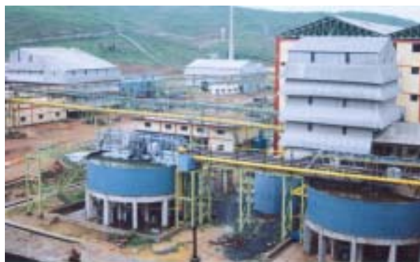
Ore processing plant, Jharkhand for UCIL commissioned by EPI
