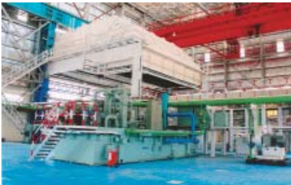
Test Bed for Frame 9 FA Gas Turbines at BHEL, Hyderabad
