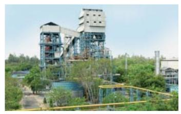
Integrated Gasification Combined Cycle Demonstration Plant, Tiruchirappalli
