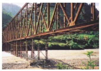
143 M Single Span Steel Bridge by TSL.
