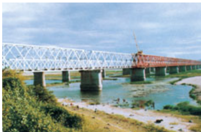
Construction of Krishna Bridge 12x90 M at Vijayawada, Andhra Pradesh by BBJ
