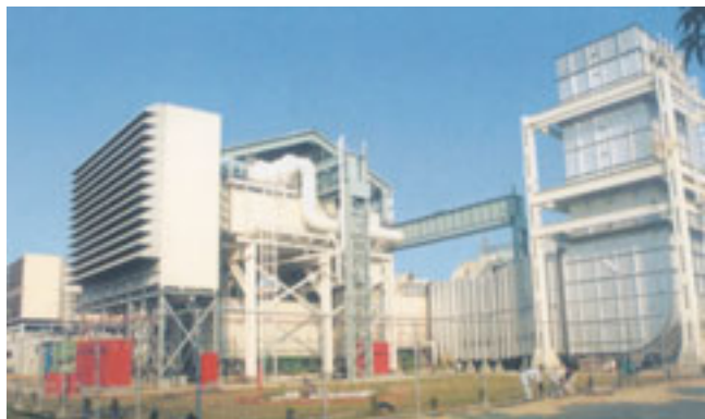
100 MW Gas Turbine-based Power Plant commissioned by BHEL on turnkey basis, at Baghabari, Bangladesh
