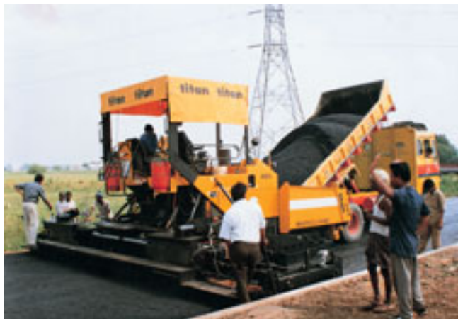
Paver Finisher with Electronic Sensor for road construction work undertaken by B & R
