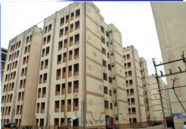
Tamilnadu Slum Clearance Board Tenements Buildings at Perumbakkam, Chennai
