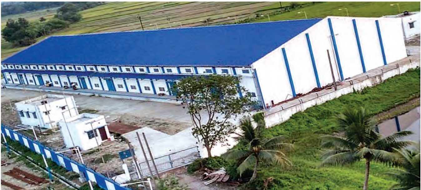
Godown Project, Diamond Harbour, West Bengal
