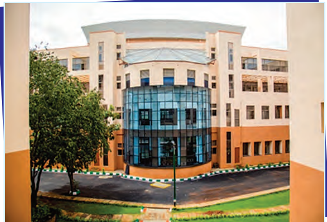
Construction of New Chemical Sciences Building at IISC Campus, Bangalore
