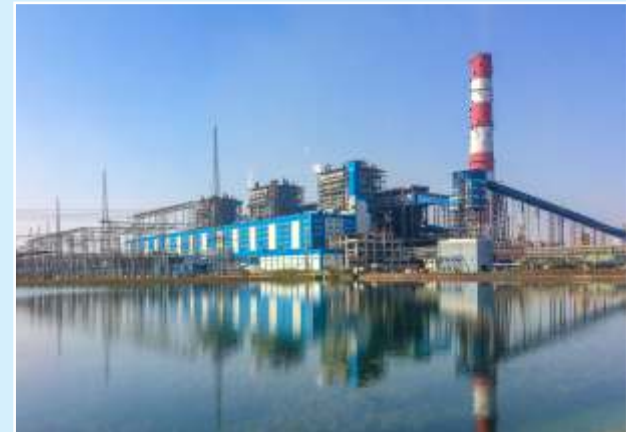
250 MW Bongaigaon Thermal Power Station
